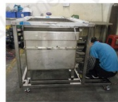
③ Tank Welding
